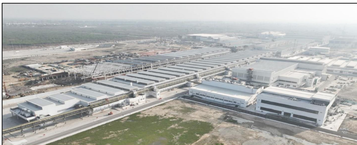
An aerial view of the first plant of Maruti Suzuki's Kharkhoda manufacturing facility
