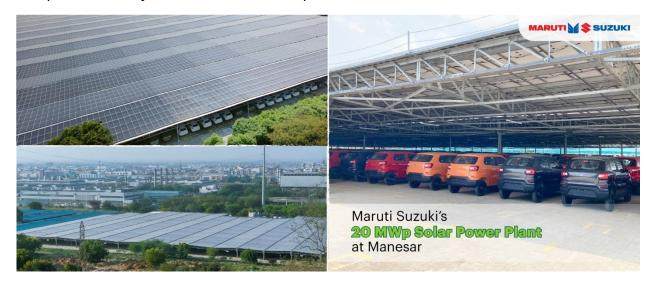
The 20 MWp car-port style solar power plant is thoughtfully designed with lowest area per unit power generation using the East-West direction concept, maximizing generation using minimum land. The facility has space to park about 9,000 finished vehicles.
