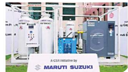
1 Ton/day Capacity Oxygen PSA Plants
