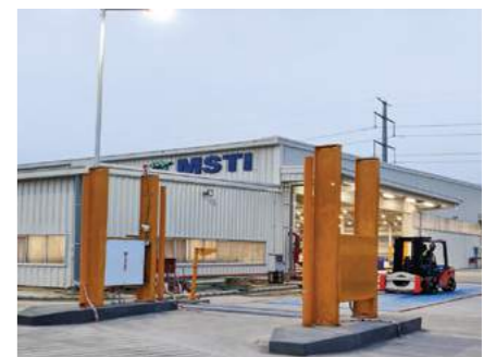
A view of MSTI facility
